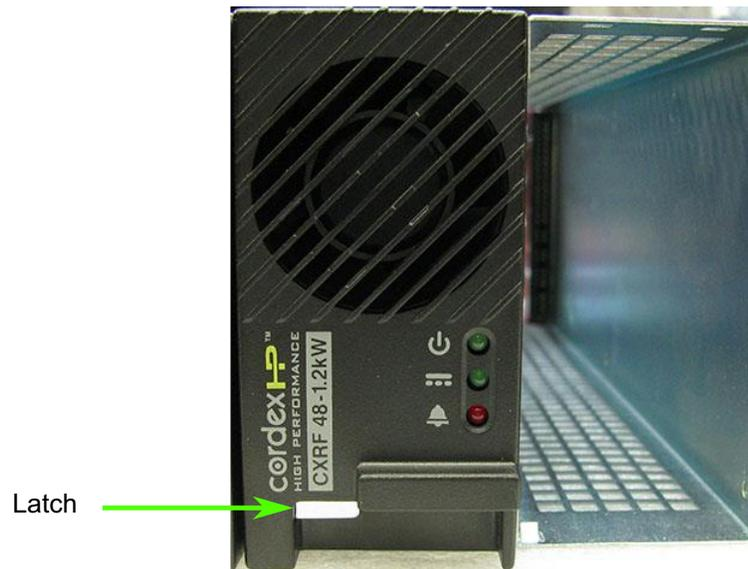
2. Place the new rectifier module on the shelf bottom and slide the module into the rear connector (inside the shelf).
