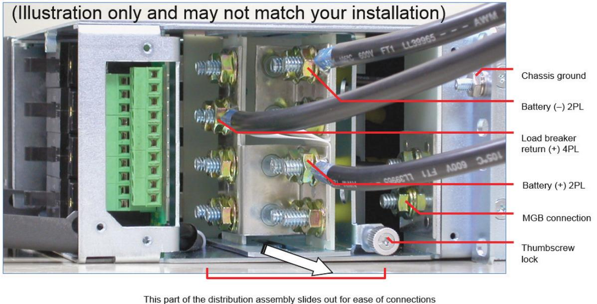
**NOTE:** Cabling must be done with enough slack to allow the distribution assembly to be locked into place.
